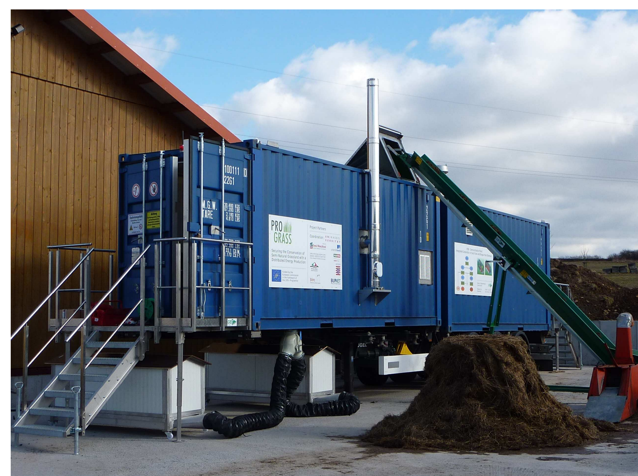
Fig. 3: Start of operation of the plant
